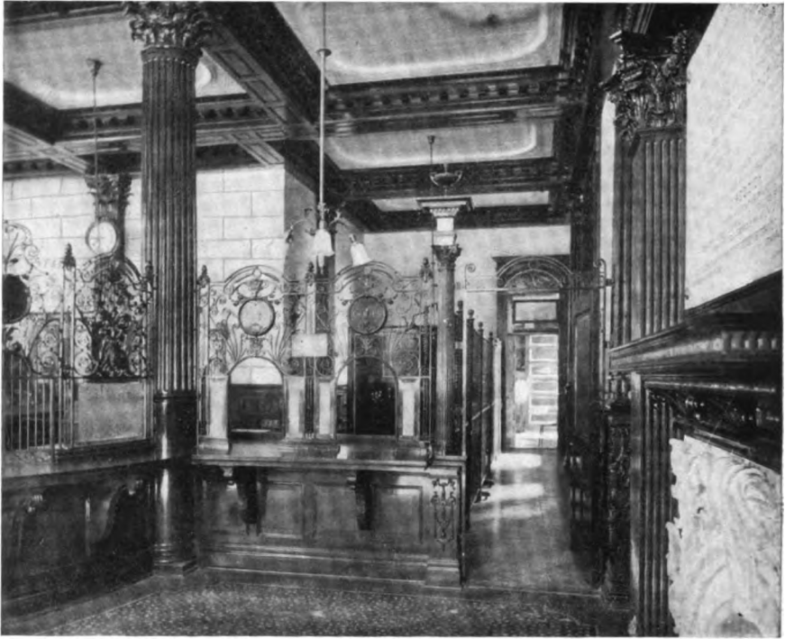
Cashier's Department and Entrance to Safe Deposit Vaults.
